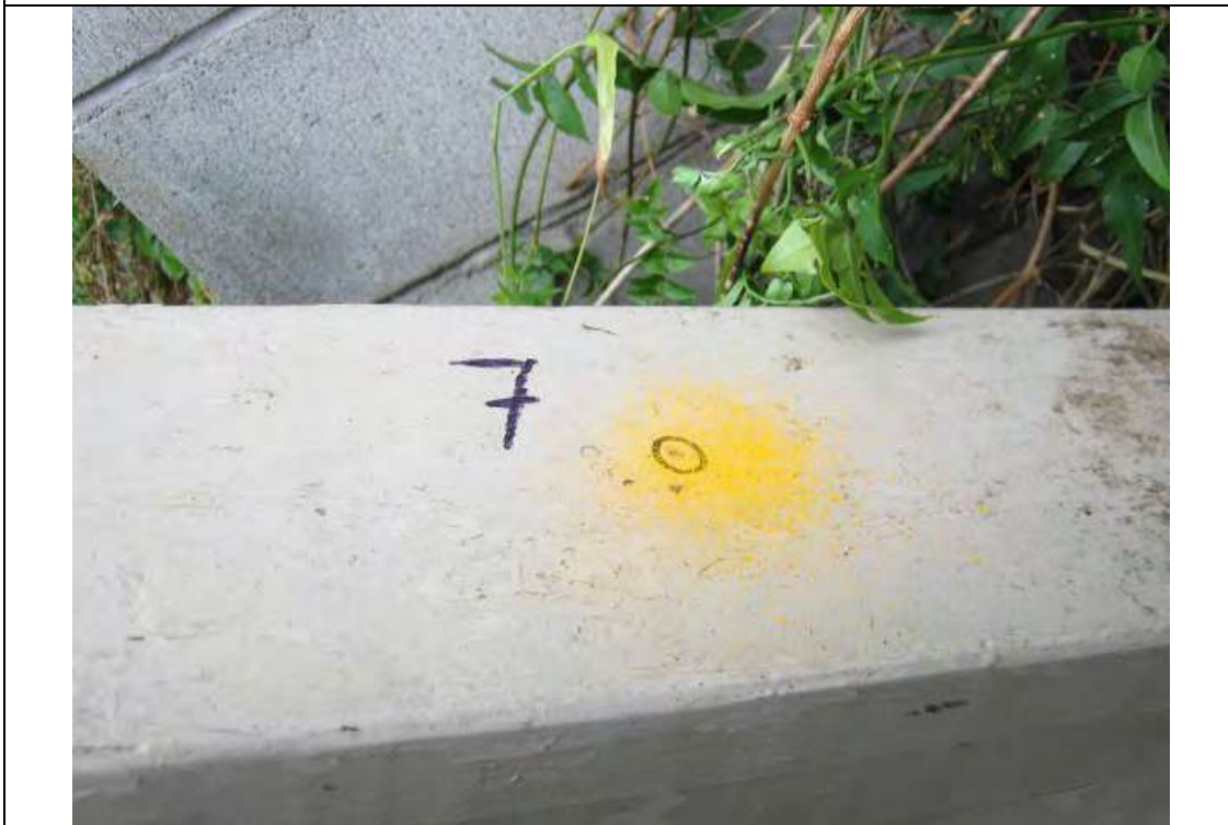
Photo showing Beam "C" and probe #7
