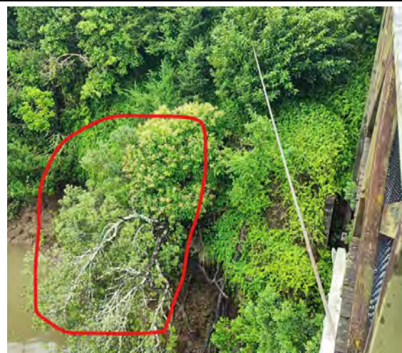
6. New slips beside the bridge on the east end
