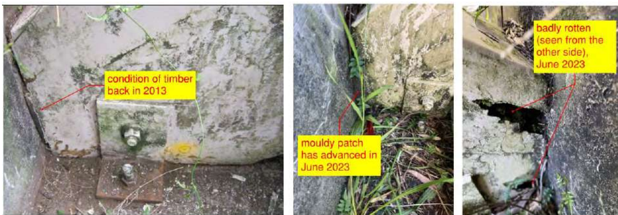
Figure 15: Side-by-side comparison of the base of the main timber arches on the Watene Rd side – Northern arches.
