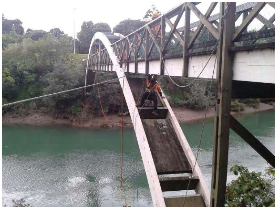
Figure 5-1 View of Inspector from west bank
