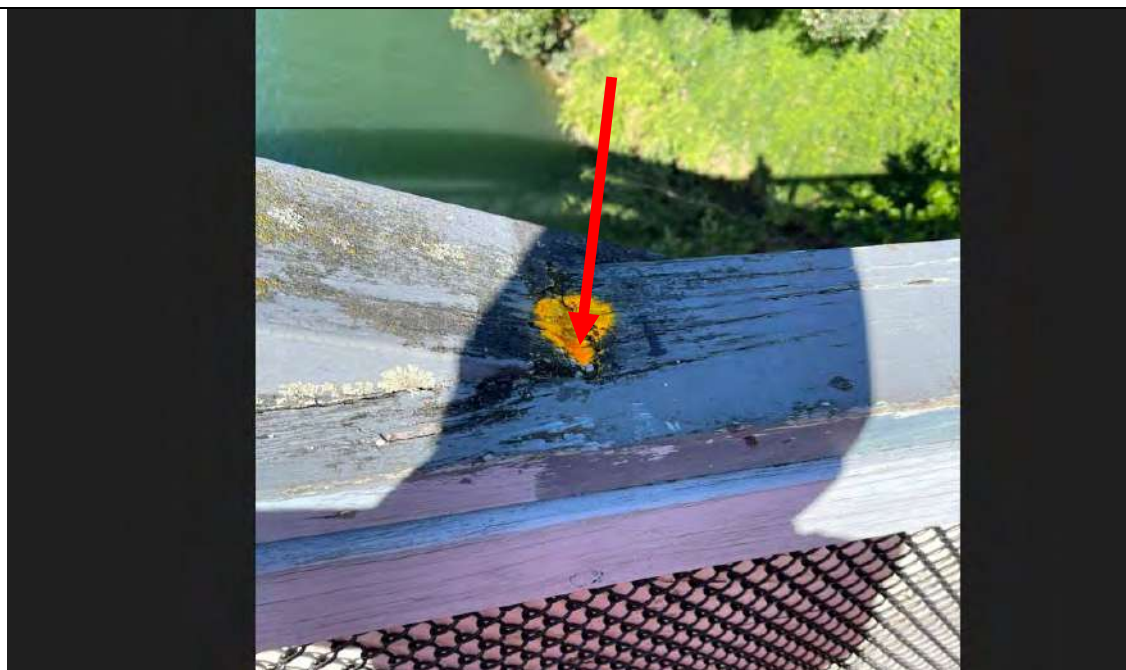
Photo showing the location of test drilling #1 The red arrow(s) depict the approximate drilling angle(s)
