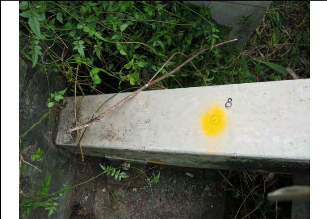
Photo showing Beam "D" and Probe #8
