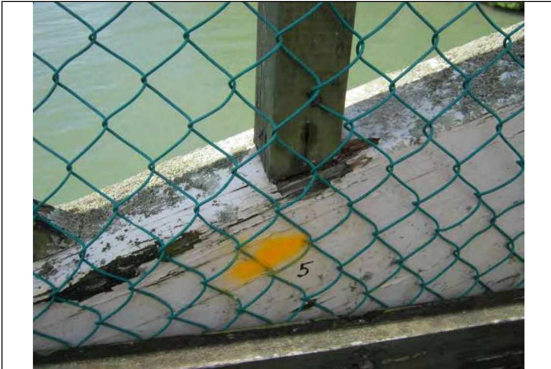
Photo showing the location of Probe #5
