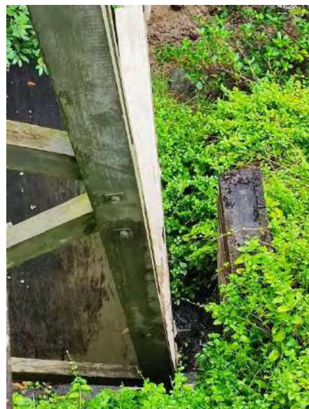
4. No erosion to the concrete footing
