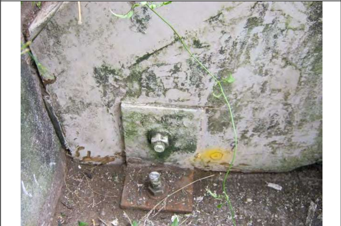
Photo showing beam "D" and probe #9
