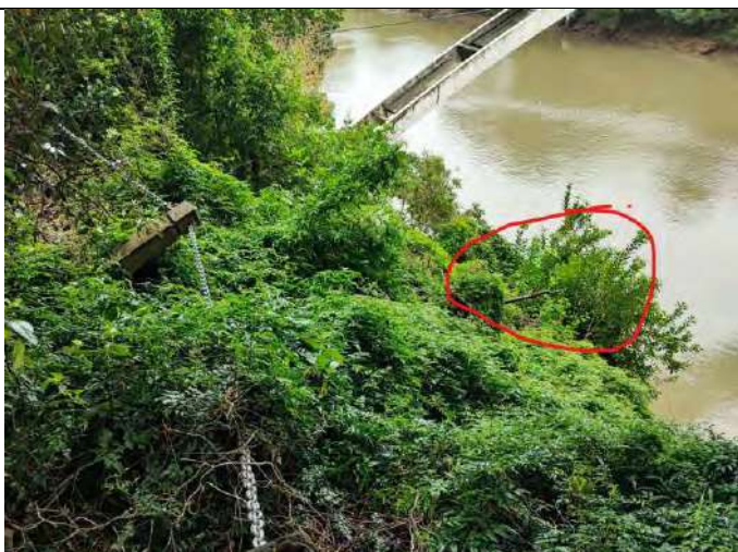
5. New slips beside the bridge on the west end
