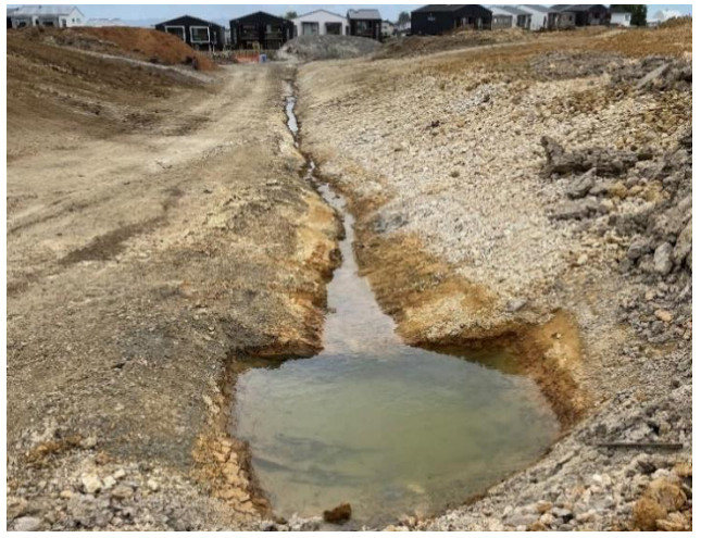
Discovery of unearthed groundwater during site earthworks.
