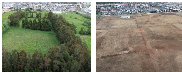
Left: Before clearing works. Right: After clearing works.
