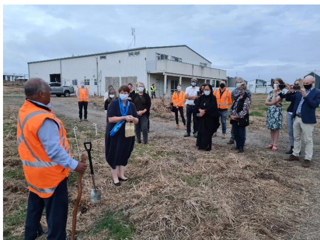
Blessing held on site with mana whenua, Upper Harbour Local Board members, HEB Construction representatives and the project team.
