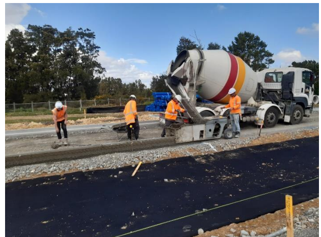
Construction of Joshua Carder Drive extension road kerbing, September 2022.
