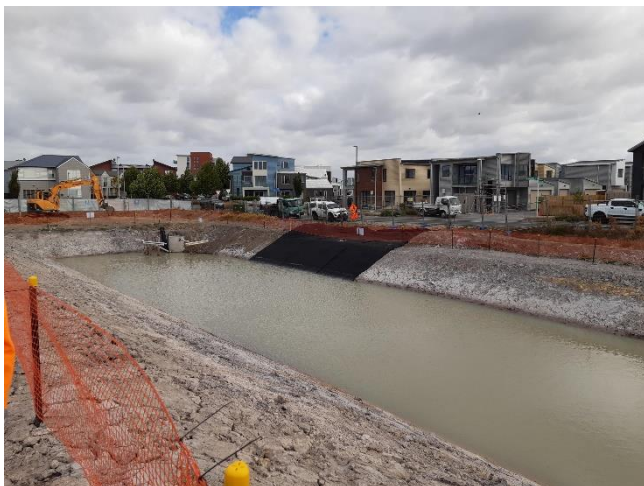
One of two temporary stormwater ponds on site.
