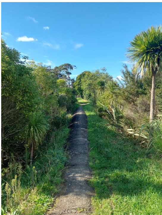
Photograph 4.3: Native vegetation either side of the Eastern Interceptor pipeline.
