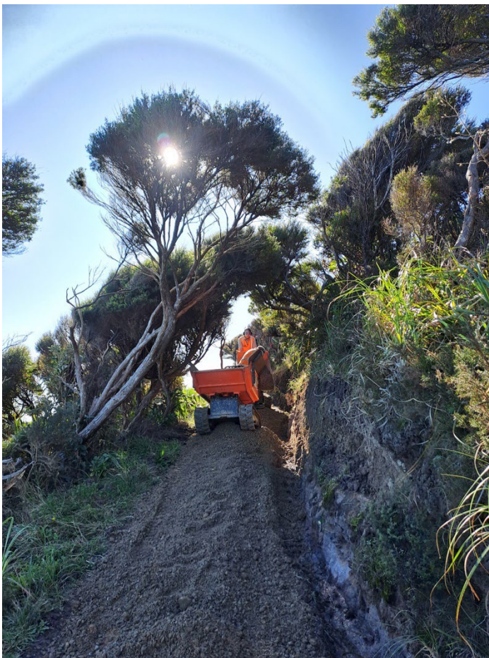
Work underway at Mercer Bay Loop track.
