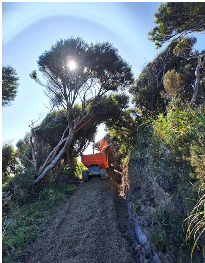
Figure 1 Work underway at Mercer Bay Loop track.
