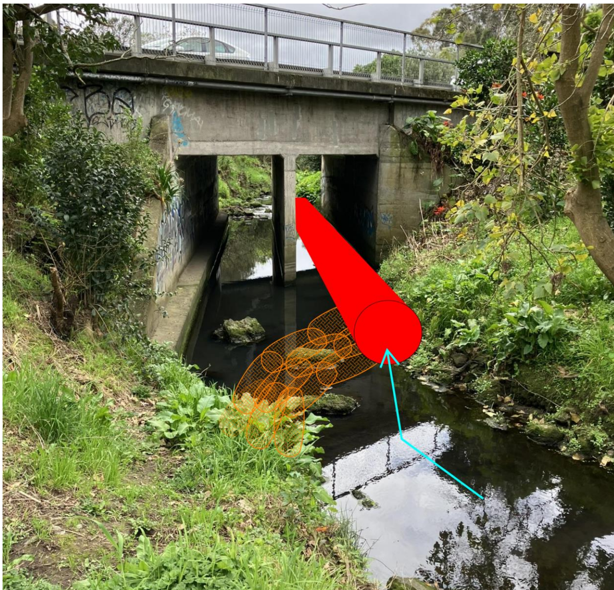
Figure 4: Diversion of creek via sandbag dam and pipe.
