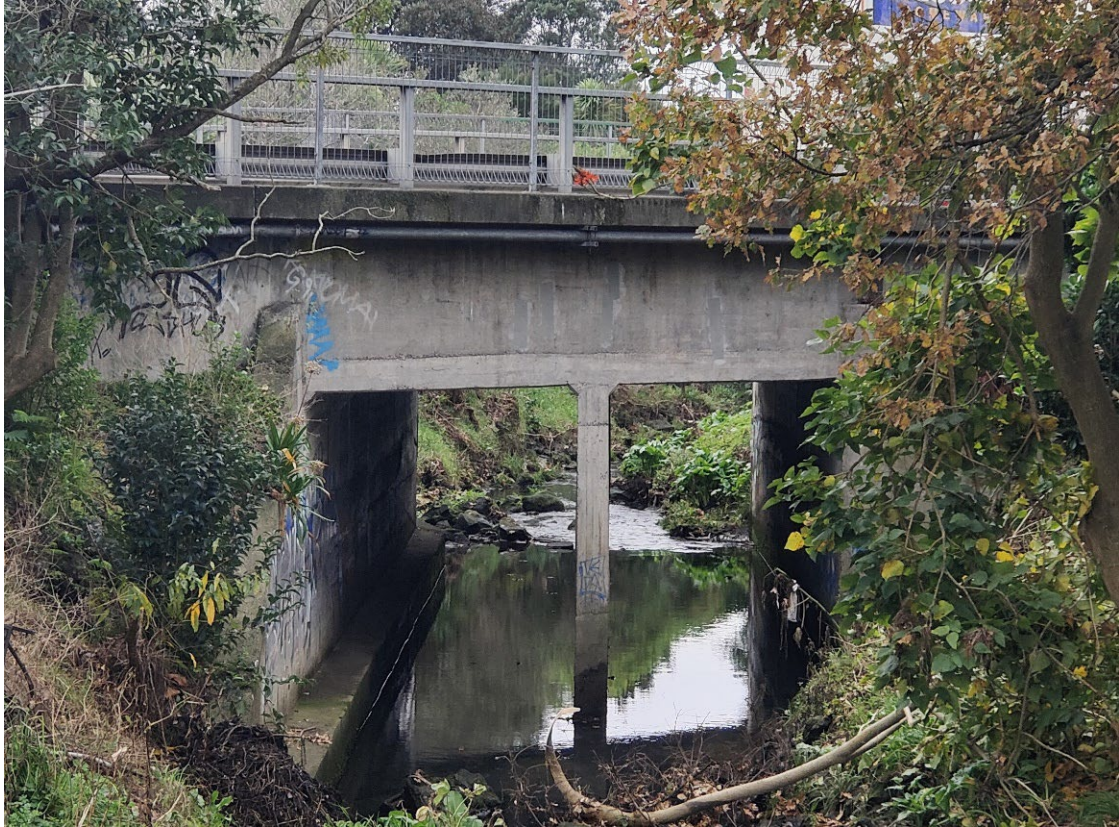
Photograph 8: The Walmsley Road bridge culvert viewed from the south.
