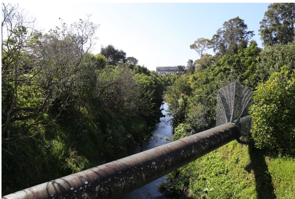
Photograph 4: View north along the Te Ararata Creek viewed from the Walmsley Road bridge Culvert, the Watercare watermain pipe bridge can be seen in the foreground.
