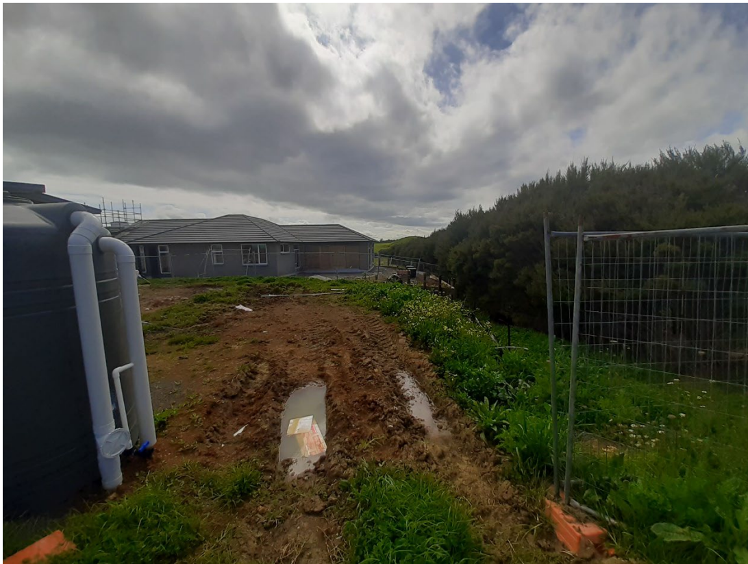
Orawahi Rd dwelling (# 8? shown) and application site to the right
