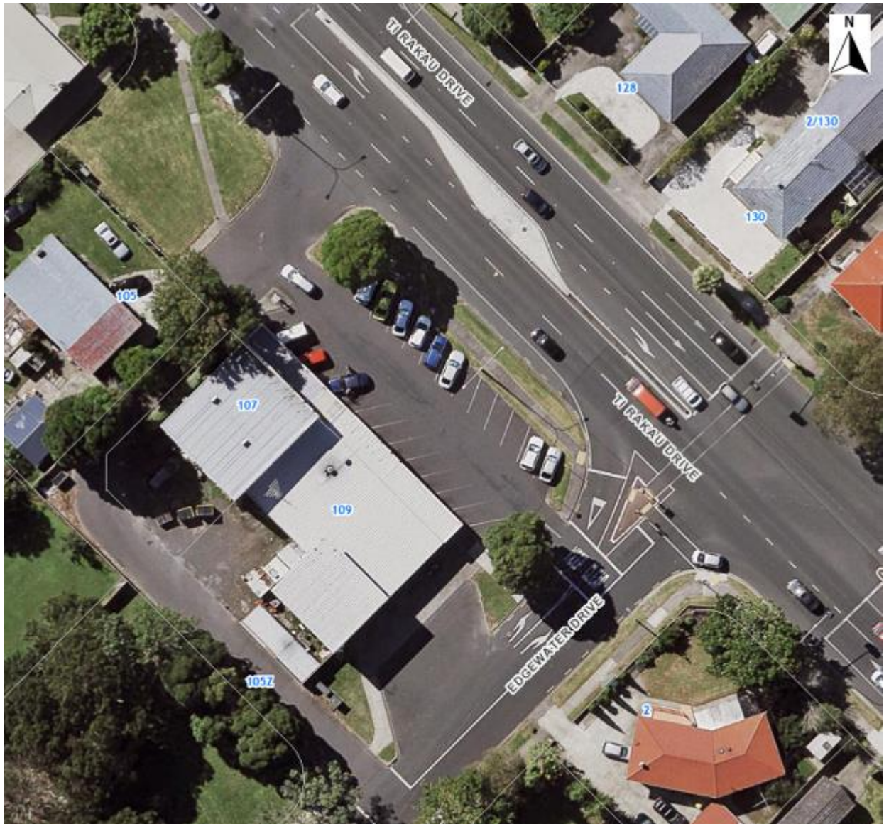
Figure 95: Edgewater Shops parking area
