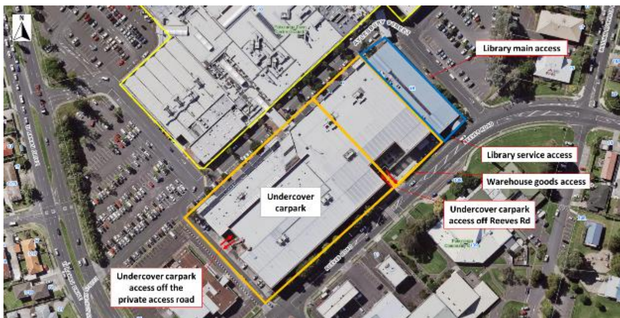
Figure 78: Pakuranga Plaza undercover carpark accesses
