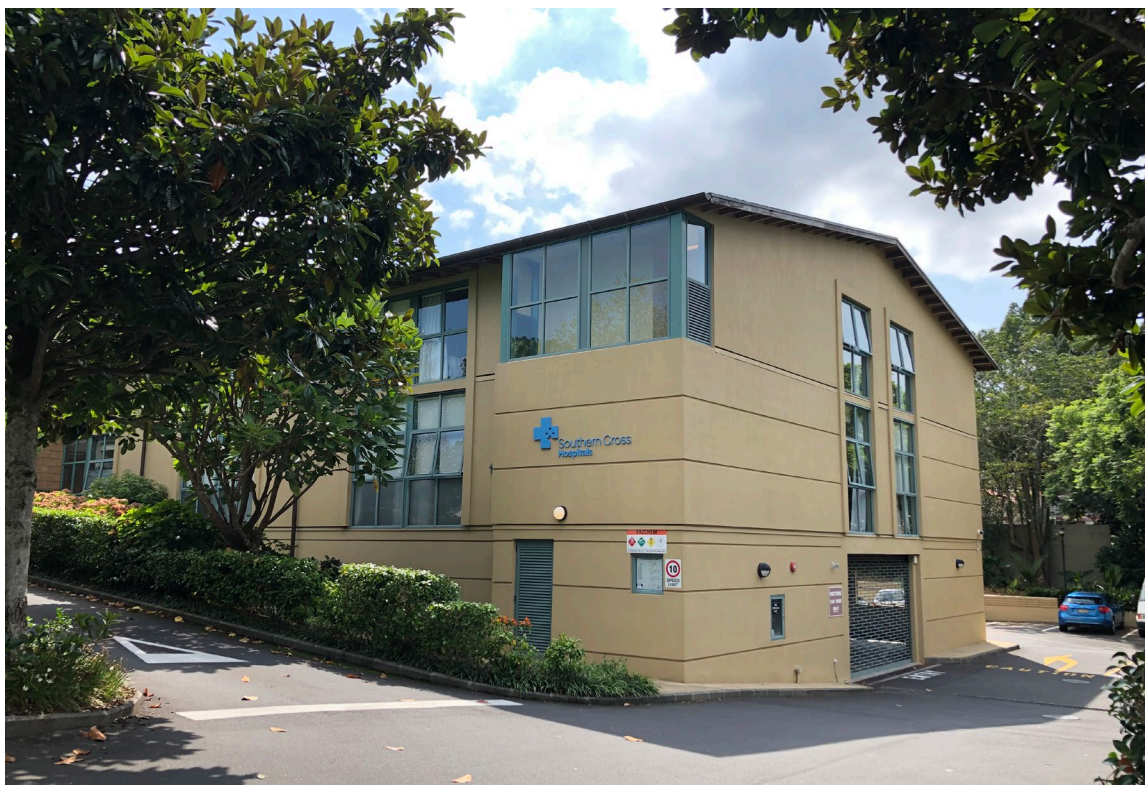
Figure 4: Existing Brightside Hospital viewed from Brightside Road
