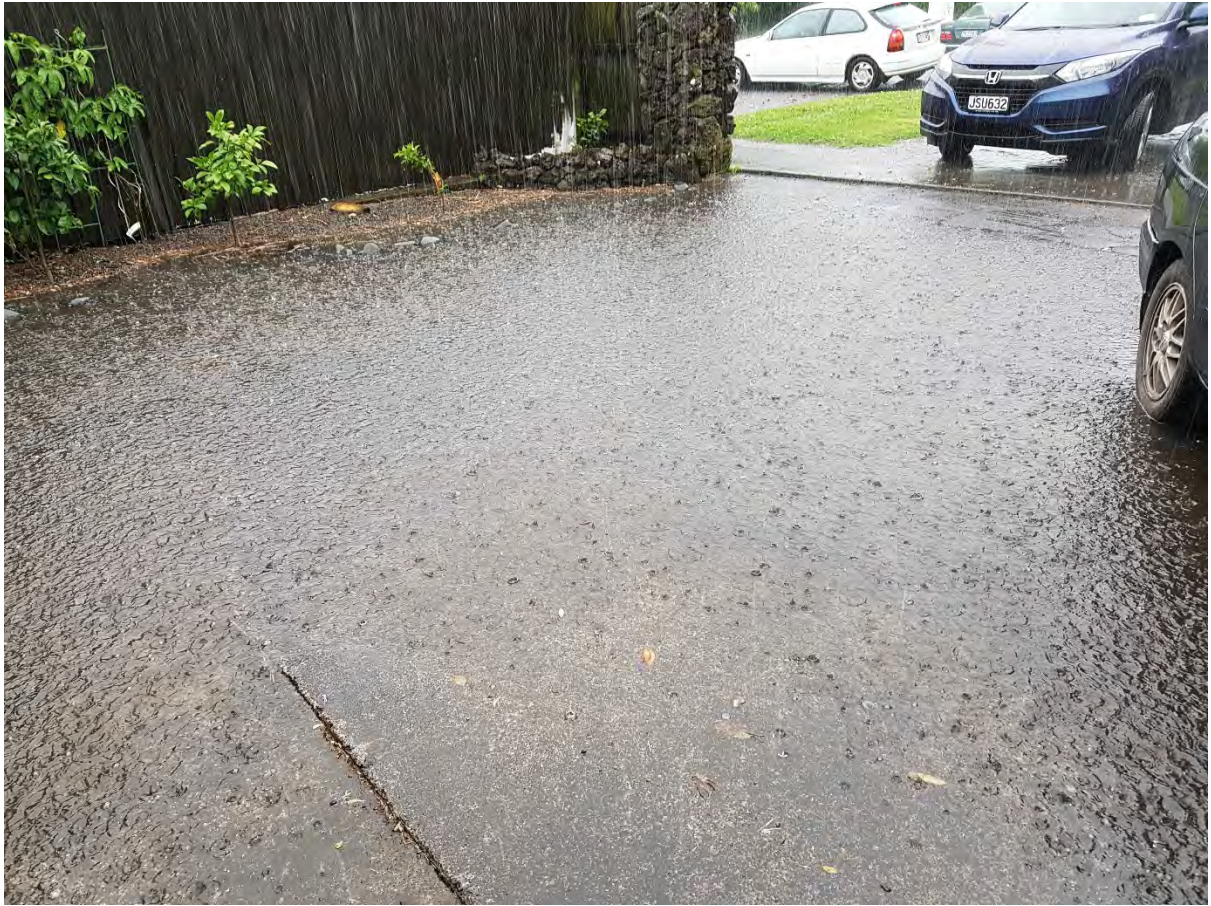
Flooding and cars moved to prevent water damage. The drain grating is under the lemon tree in the centre of the picture and is obviously completely useless in this downpour.
