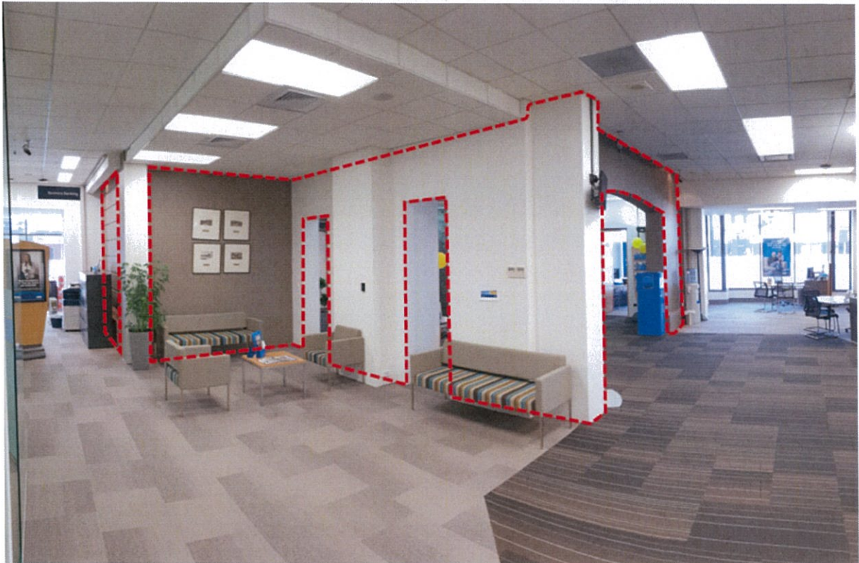
Photo 1 – Internalised external walls, looking south east
