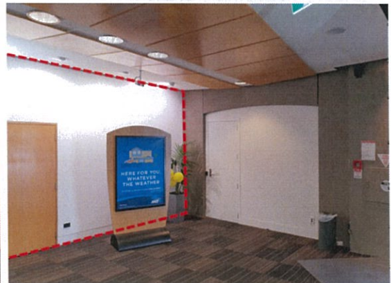
Photo 2 – Internalised external walls, looking north
