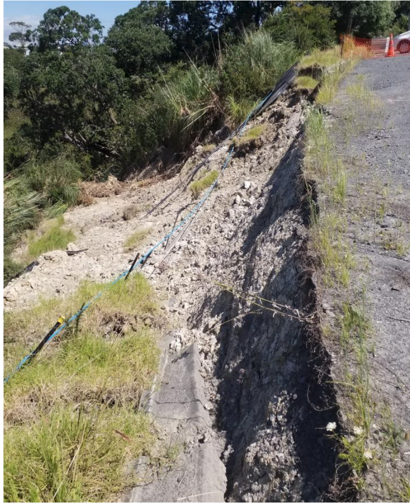
Figure 10: At least 2m of land has been lost from the top of the slope
