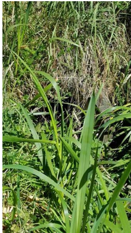
Figure 13: Culvert observed at/near the recorded location of the timber water retention feature/slucice CHI 18372
