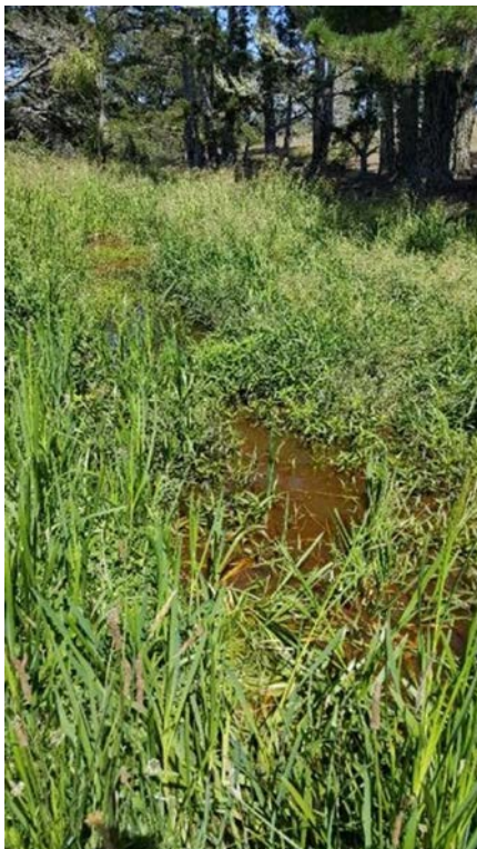
Figure 12: Showing the general condition of the watercourses south of the Baker Lane alignment where the timber water retention feature/slucice CHI 18372 was recorded; looking north
