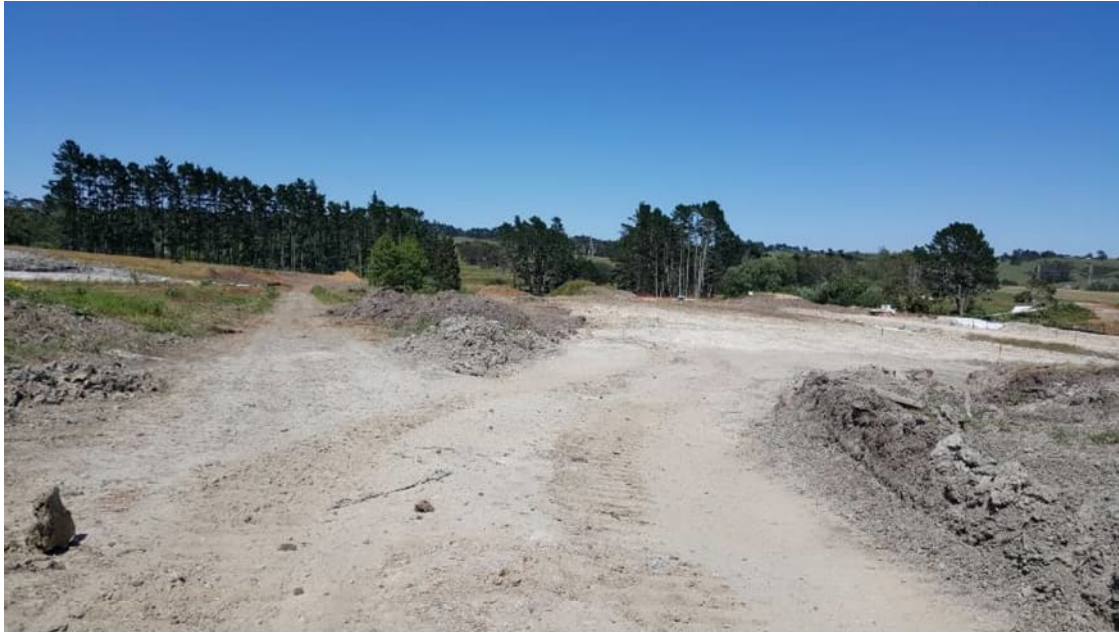
Figure 11: Photo taken from within the Baker Lane development, looking south-west over proposed Baker Lane alignment
