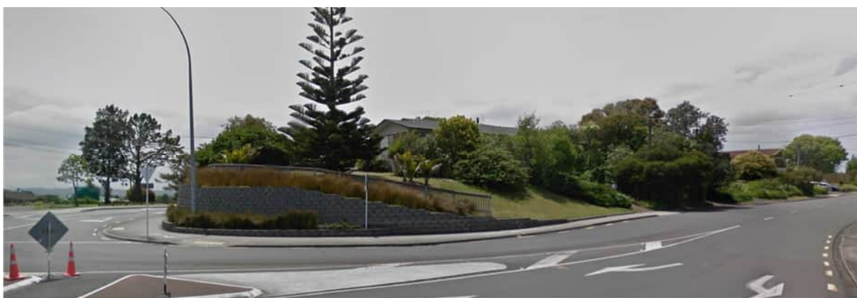
Figure 7: Existing retaining wall feature and buffer planting at Don Buck Road / Royal Road intersection
