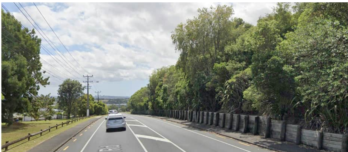
Figure 6: Existing timber retaining wall and buffer planting at Don Buck Road / Royal Road intersection
