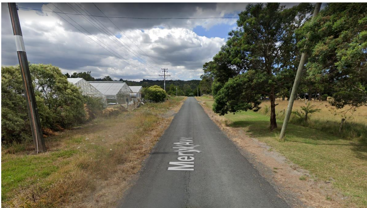
Figure 7-12: Meryl Avenue – Existing Form (View North at 29 Meryl Avenue)
