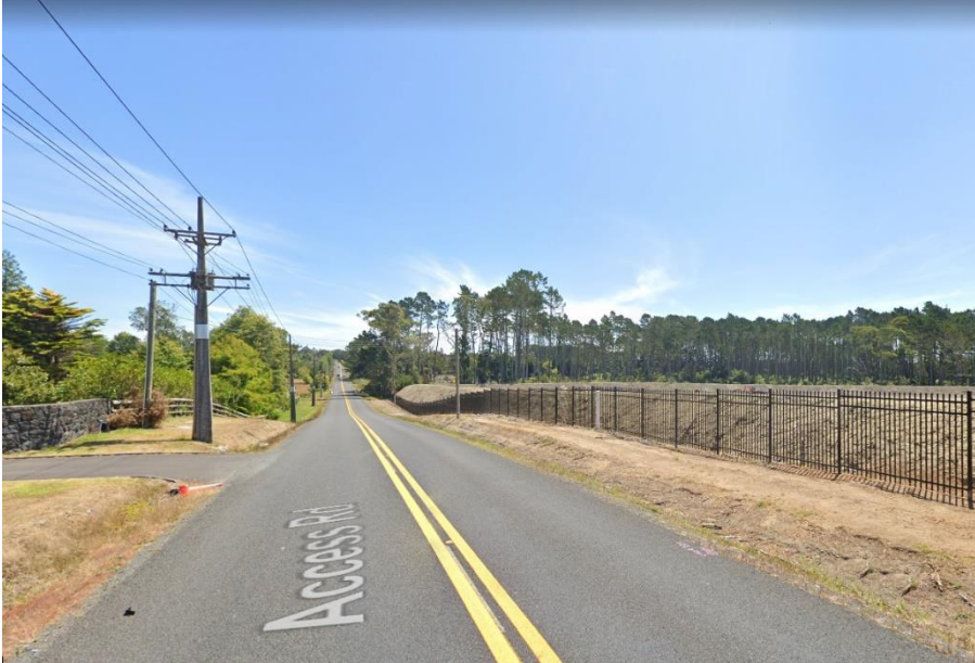
Figure 8-5: Existing Access Road Corridor (Rural Section)
