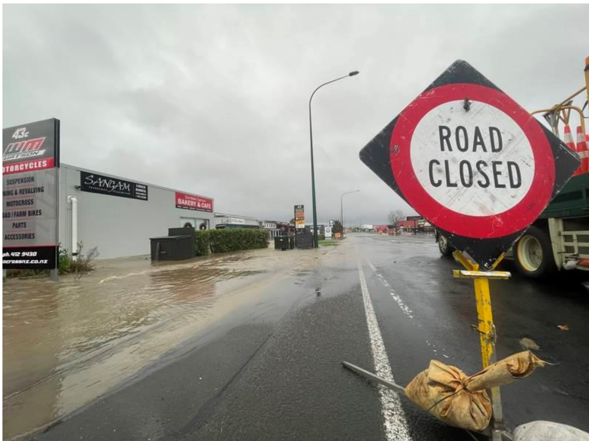
Figure 3-1 Flooding closed the main road in Kumeū. (Source: 1 NEWS)
