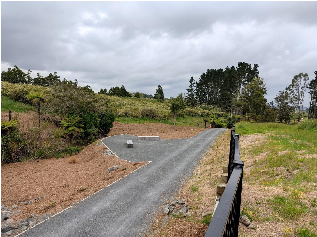
Figure 39: Modern modification close to the crossing of Waiarohia Stream.
