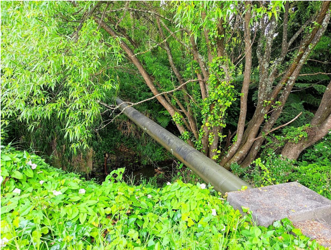
Figure 25: View over stream crossing looking downstream.
