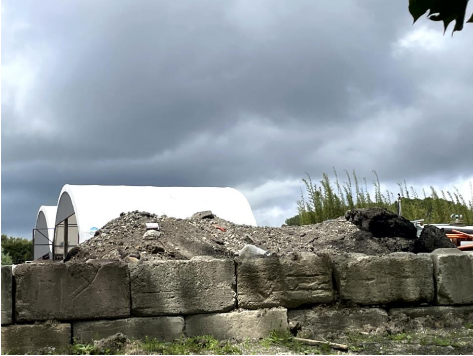
Fig1-3 construction work on 5 speeding road
