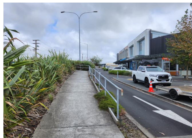
Hobsonville Road slip road entrance (one way) with pedestrian link and access ramp with safety barrier.
