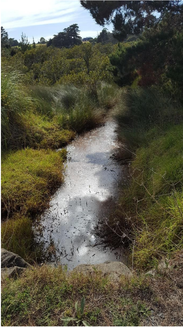
Figure 9: View of stream feeding into western culvert
