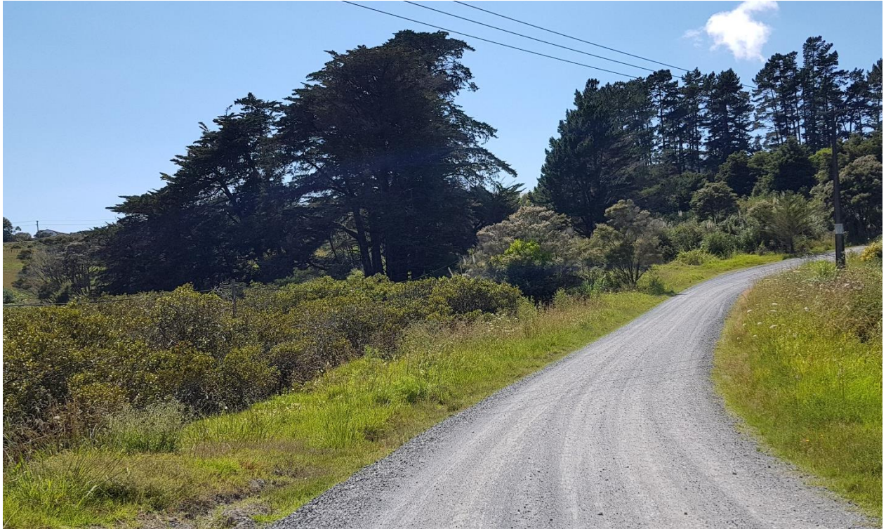
Figure 7: Existing WWTP access road looking east over eastern culvert.
