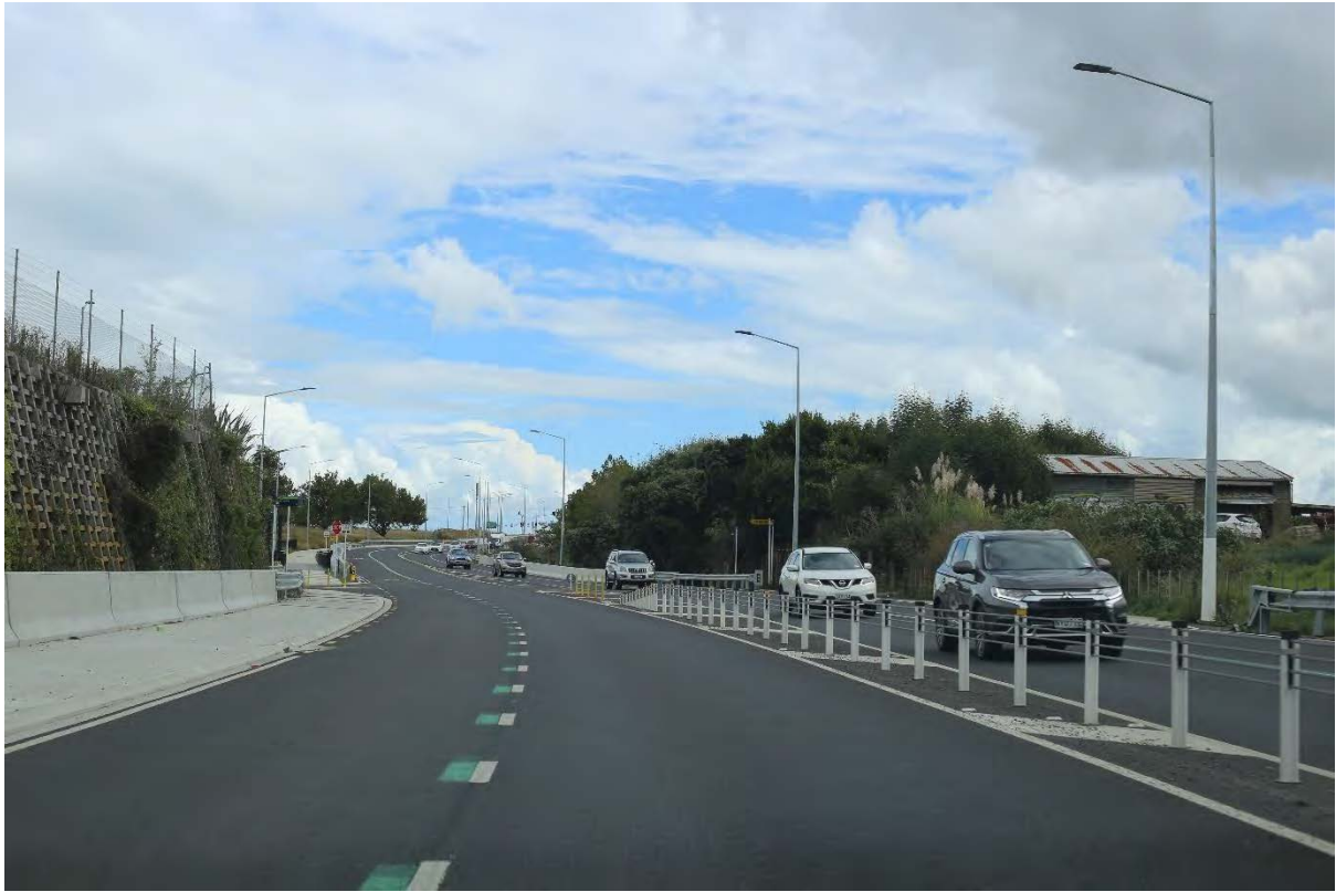
Figure 37: Puhinui Road (SH20B) looking east from Prices Road
