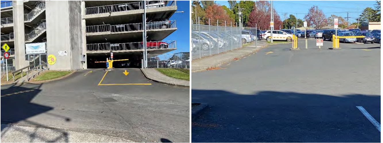
Figure 5-4: Current at grade and multi storey main car park entrances to be relocated
