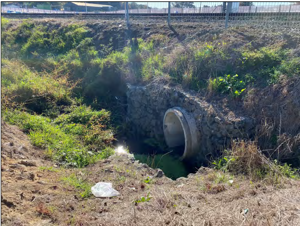
Figure 4-15: Culverts at Middlemore Station
