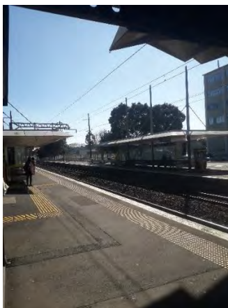
Photo 2 – Middlemore Station existing platform area, looking north
