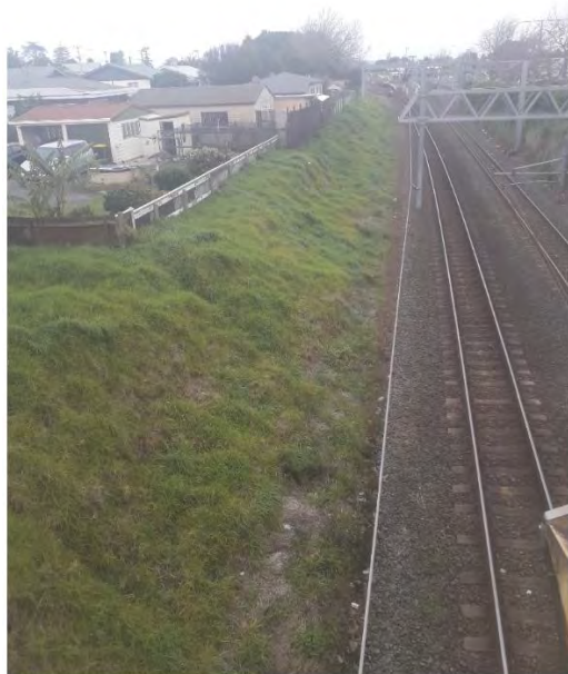
Photo 5 – looking north to Papatoetoe Station – area of new retaining wall
