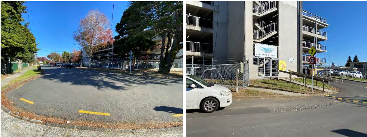
Figure 3-8a and b: Orakau Road looking south from the cul-de-sac and Orakau Road from Middlemore Station looking west to car park entrances and drop off area
