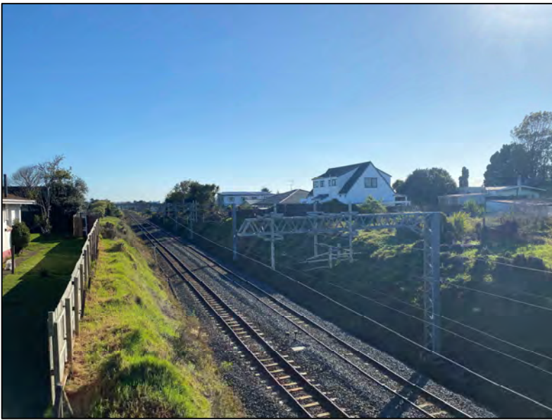
Figure 4-10: View North from Bridge Street
