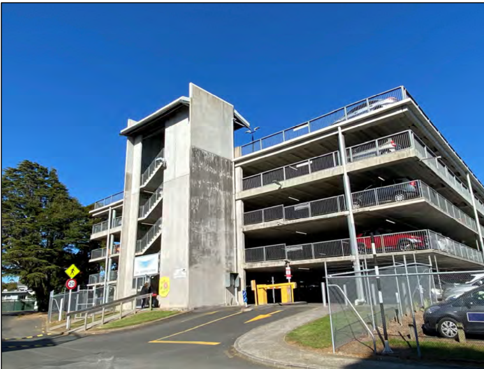
Figure 4-4: Multi-storey car park for hospital staff
