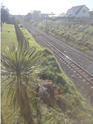
Photo 6 – looking north, Bridge St Papatoetoe – area of new retaining wall
