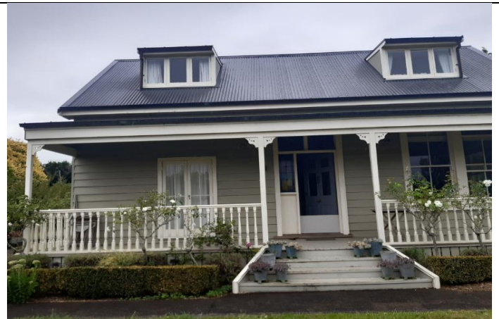
Figure 14: Front (eastern) elevation of residence. AC, 10 February 2021.
