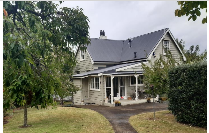
Figure 12: Side (southern) and rear (western) elevations of residence. AC, 10 February 2021.
