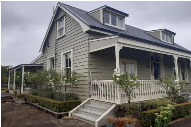
Figure 13: Front (eastern) and side (southern) elevations of residence. AC, 10 February 2021.
