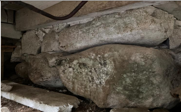
Figure 11: Two layers of boulders in the vicinity of the current fireplace. AC, 10 February 2021.
