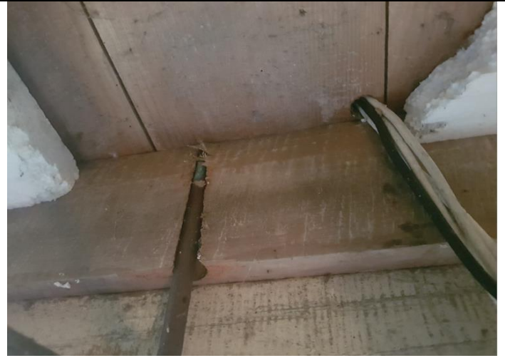
Figure 10: Approximately 210mm floorboards visible, suggest this area of the building has an early date of construction, aligning with a late 1850s date of construction. AC, 10 February 2021.
