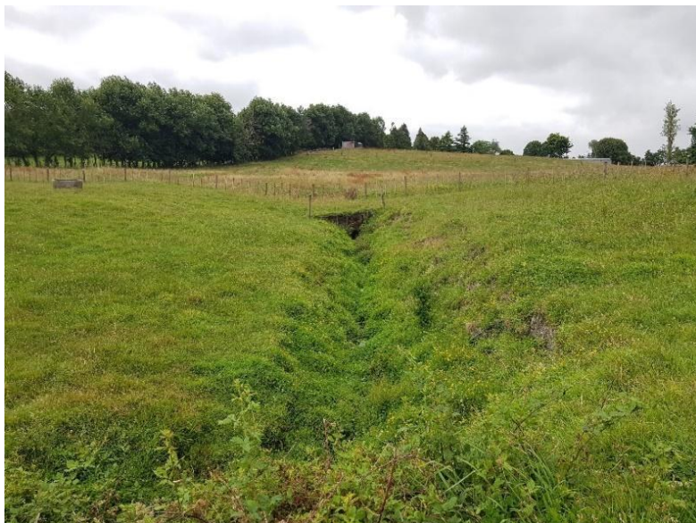
Photograph 3.1: View into Stream A headwaters. Perched culvert shown, downstream of the two upper branches of Stream A.
