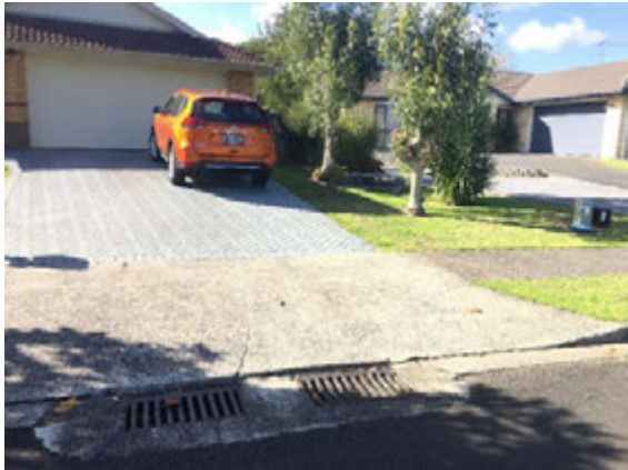
Photo 1 and 2 – Double catchpits and Large inlet device, 6 Beverage Place, Papakura
