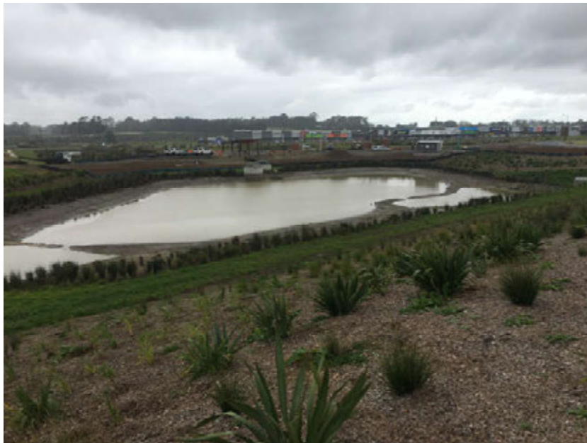
Typical Wetland for Development
