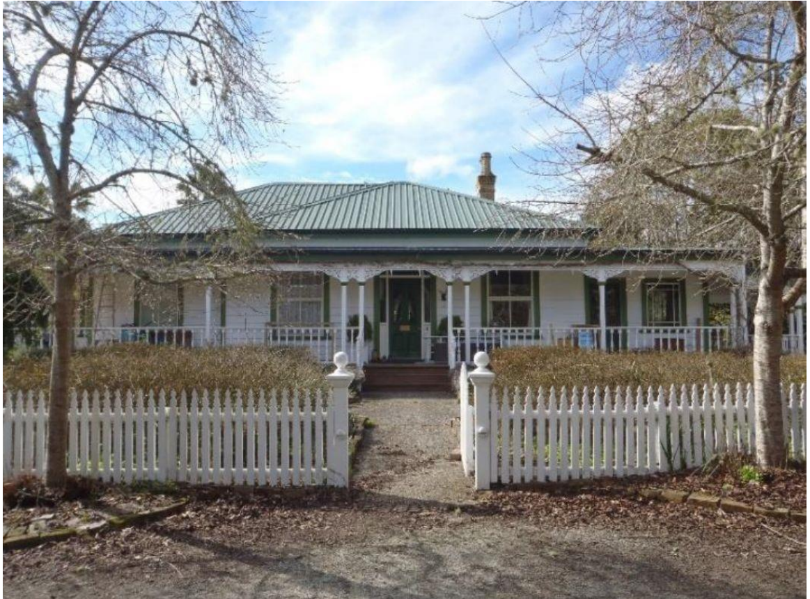
Figure 3. View of the entrance to the residence. Source: Jones and Phear 2016
