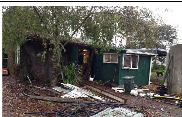
Photo 14: Workshop, facing north west.
