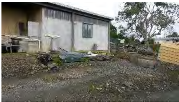
Photo 3: The redundant cow shed, facing south.
