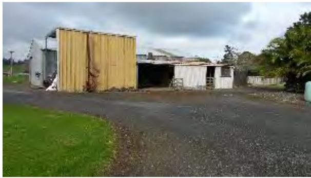
Photo 1: The workshop, facing south.
