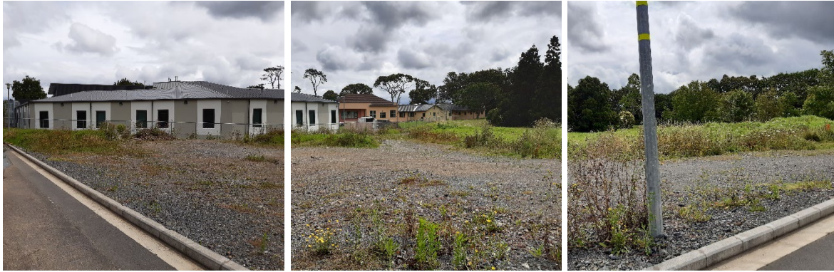
Figure 6: Photos of Northern site, from internal road boundary with 1 Carrington Road. Source: Elisabeth Laird, site visit 12 January 2023.
