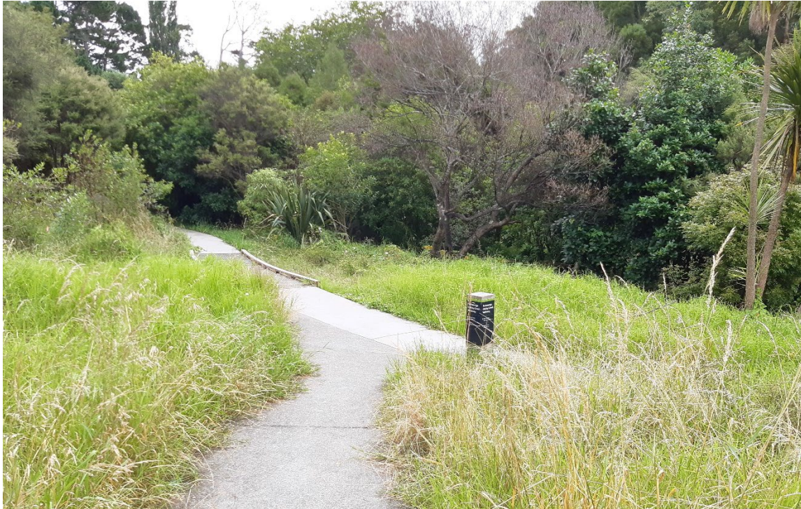
Figure 11: Connection of new path to Te Auaunga walkway. Source: Elisabeth Laird, site visit 12 January 2023.
