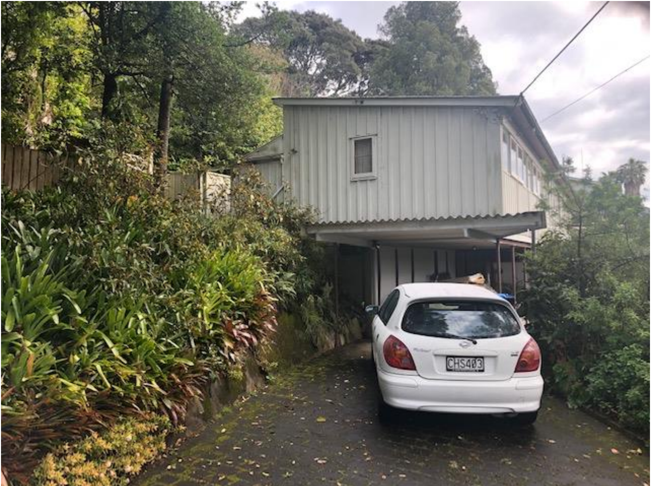
Figure 1: 10 Scherff Road, Remuera (Auckland Council 2019)
