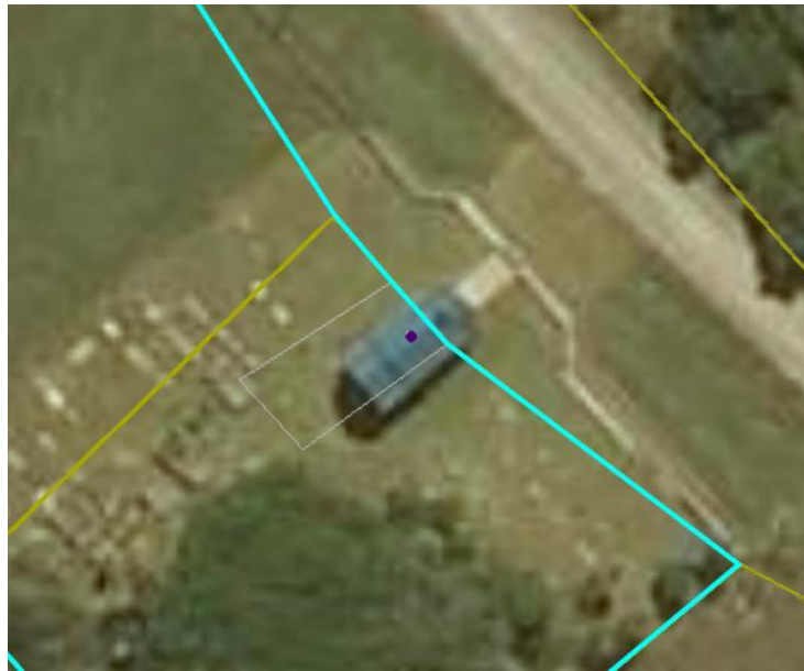
Figure 3: 67 Shegadeen Road, Wharehine, with the blue line showing the property boundary
