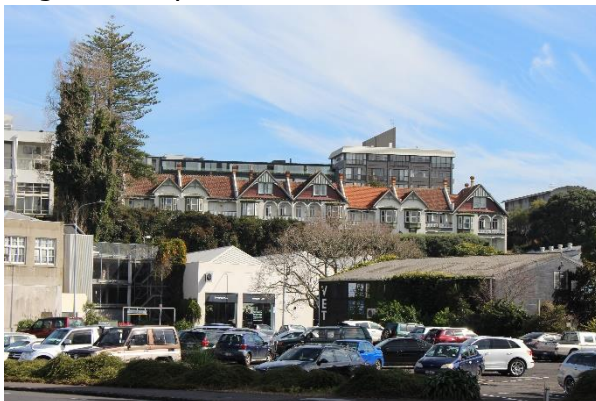
View from the Strand, looking SW
