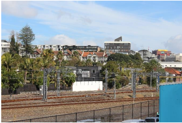
Quay St looking SW
