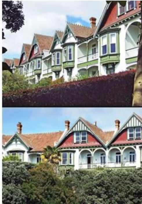
Dilworth Terrace Houses. Image courtesy of www.flickr.com .
