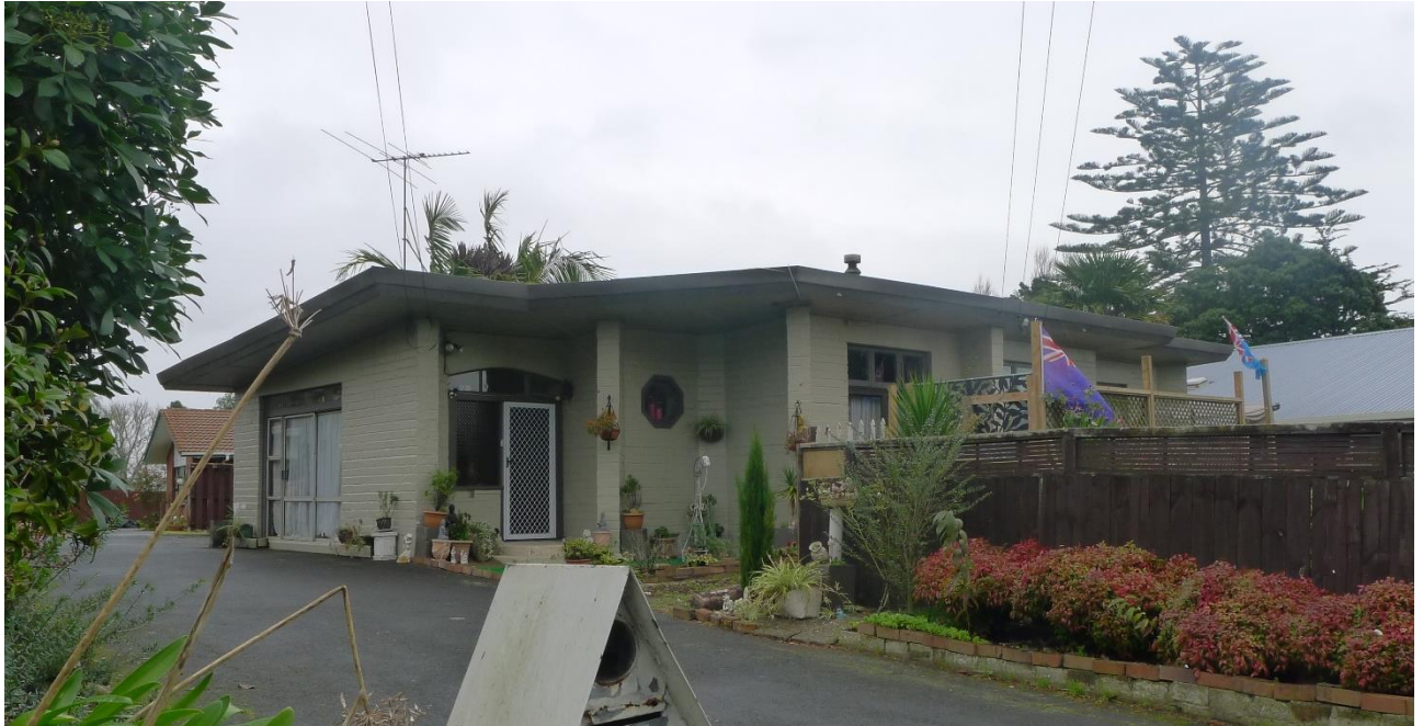
Figure 17: Residence, 1/11 Alfriston Road (Auckland Council, 9 June 2016)
