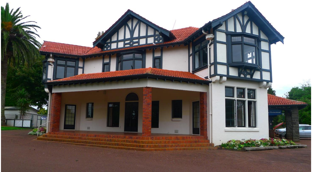
Figure 7: David Nathan Park, 68R Hill Road, Hill Park (Auckland Council 2016)
