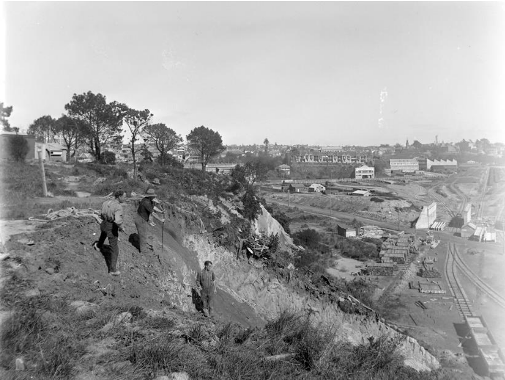
Figure 7. The view from Campbell's Point, looking W, in 1926 showing reclamations of St Georges bay and Mechanics Bay, with Dilworth Terrace Houses (centre) (Sir George Grey Special Collections, Auckland Libraries, 4-3960)
