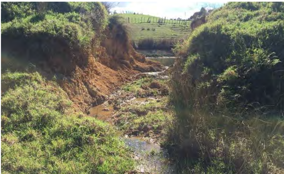
Figure 32: View of pond draining into upper permanent section of Watercourse I.
