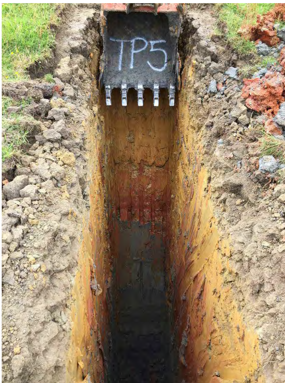
TP05-19 – TEST PIT EXCAVATION
