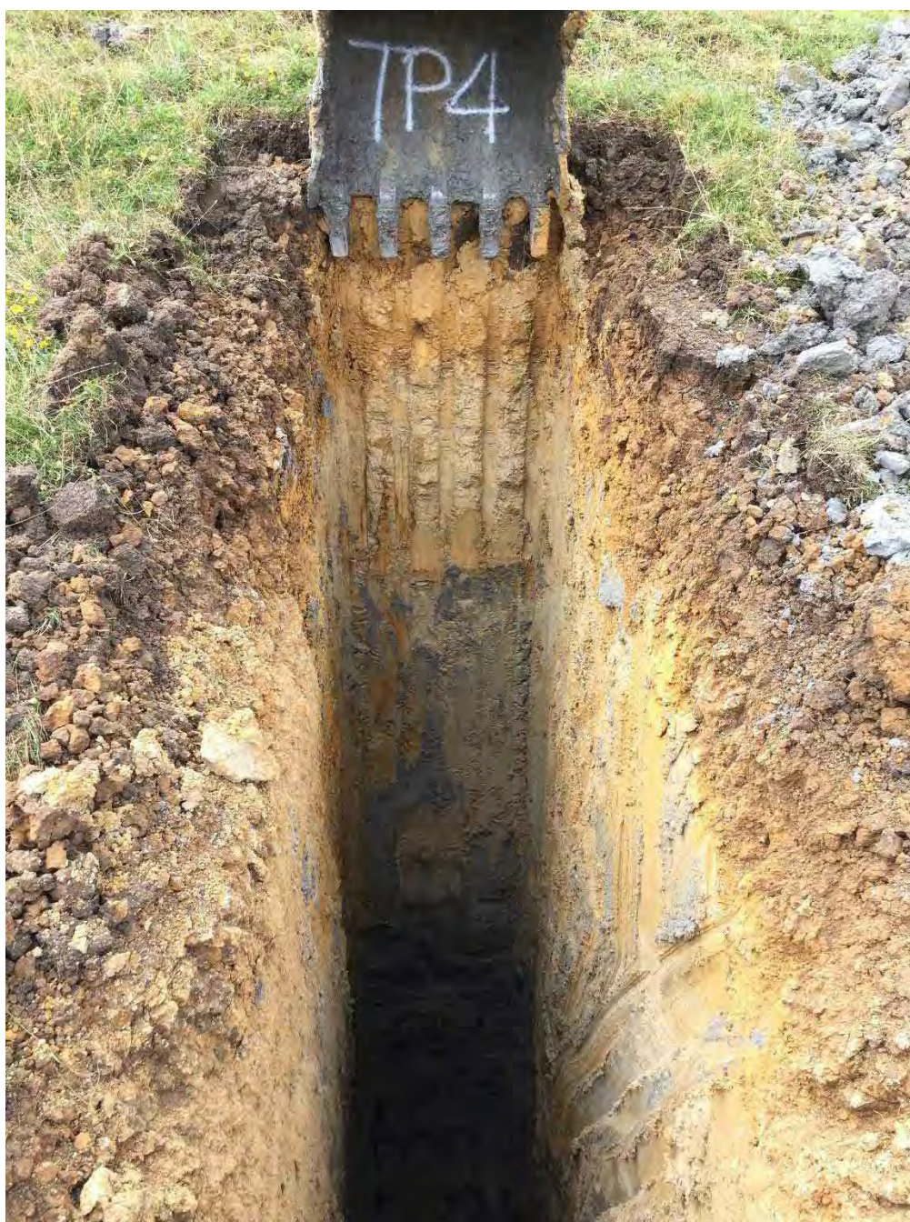
TP04-19 – TEST PIT EXCAVATION
