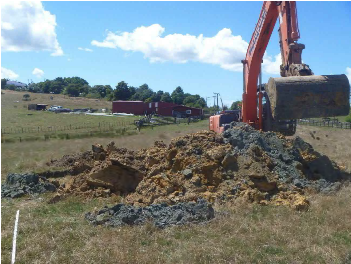
TP215 – Spoil pile
