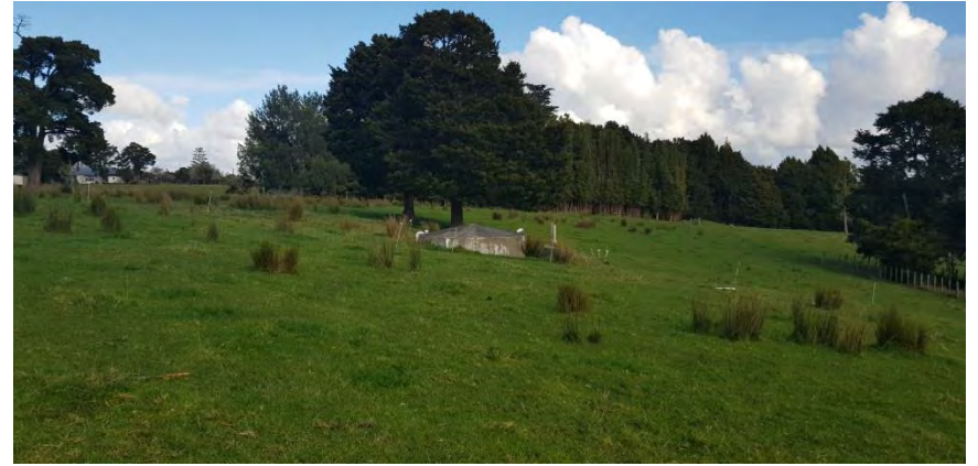
Septic Tank in Western Area
