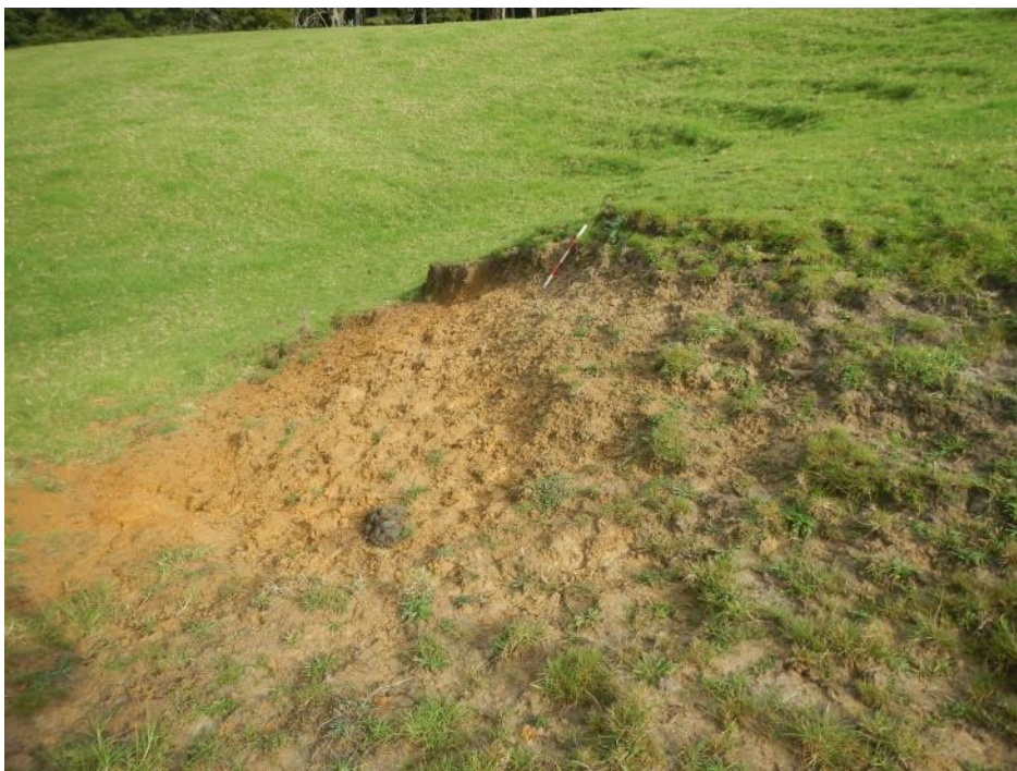
Figure 47. Example of exposed soil profile caused by cattle pugging/wallowing
