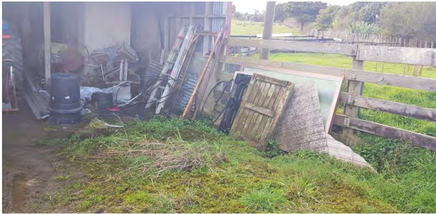
PACM sheeting outside Shearers Shed
