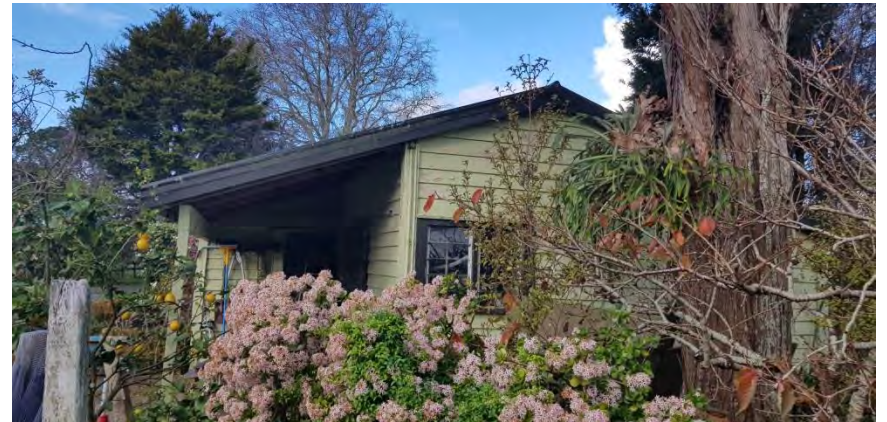
Garage (PACM Soffits)
