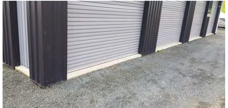
Concrete Lined Large Garage
