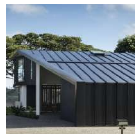
PROFILED METAL ROOFING & WALL (WRAPPED) (CHARCOAL GREY)
