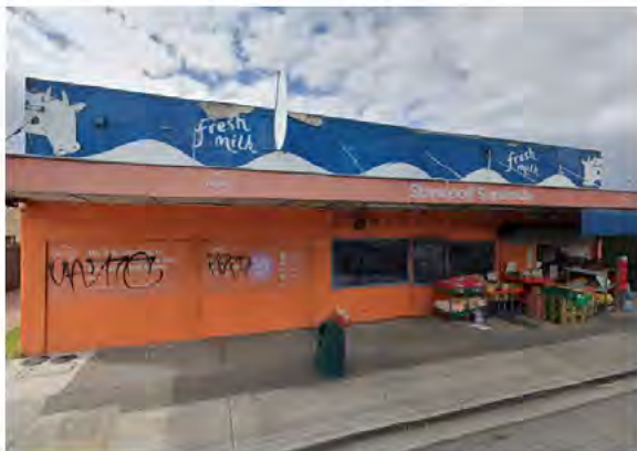
Sharland Superette, Mangere East (‘Fresh Milk’ exterior wall wrap and ‘Skinny’ orange building colour)
