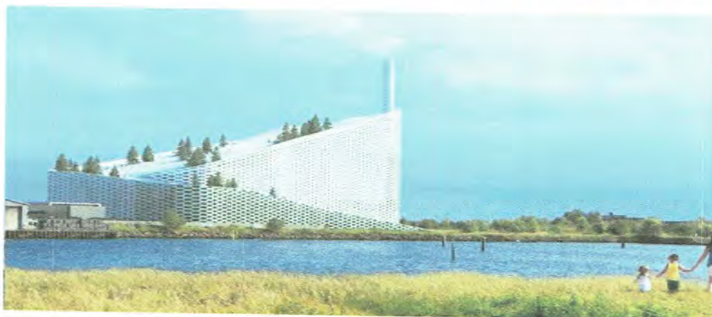
A waste to energy plant in Denmark, designed engineering company Ramboll.
