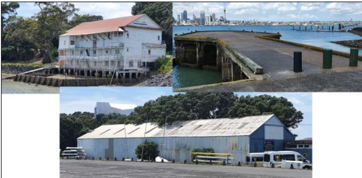
Figure 7: Takapuna Boating Club building, old wharf, Takapuna Rowing Club building.
