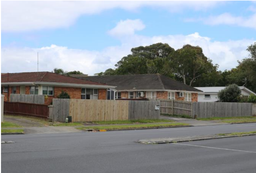
Figure 6-5 Typical Housing on Ti Rakau Drive
