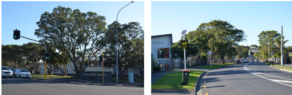
Figure 29: St Thomas's School, on the corner of Kohimarama Road and Allum Street. The image on the left illustrates the corner frontage and that on the right, the Kohimarama Road frontage.
