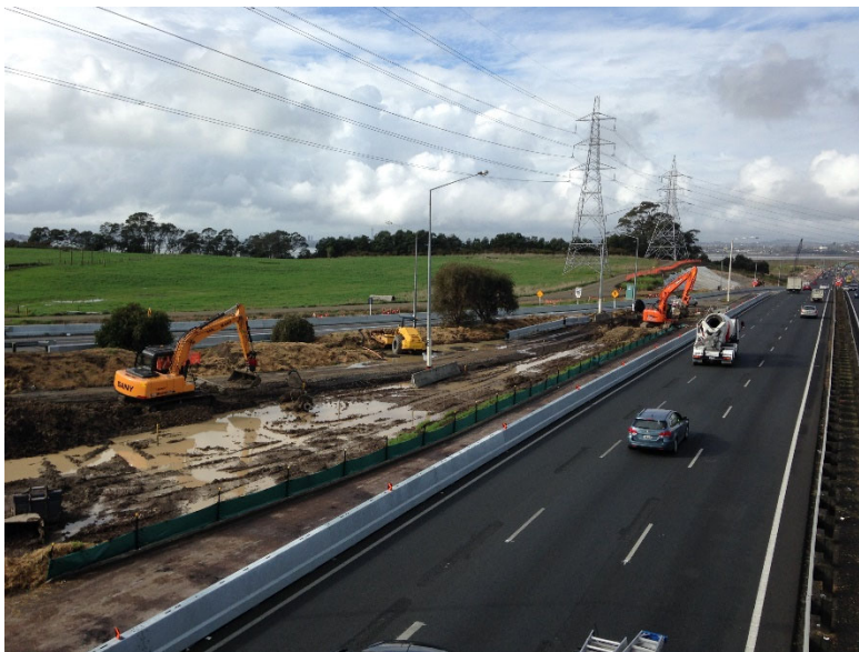
Photo 3: Silt Fences used to treat construction water, used on the North-Western Motorway.
