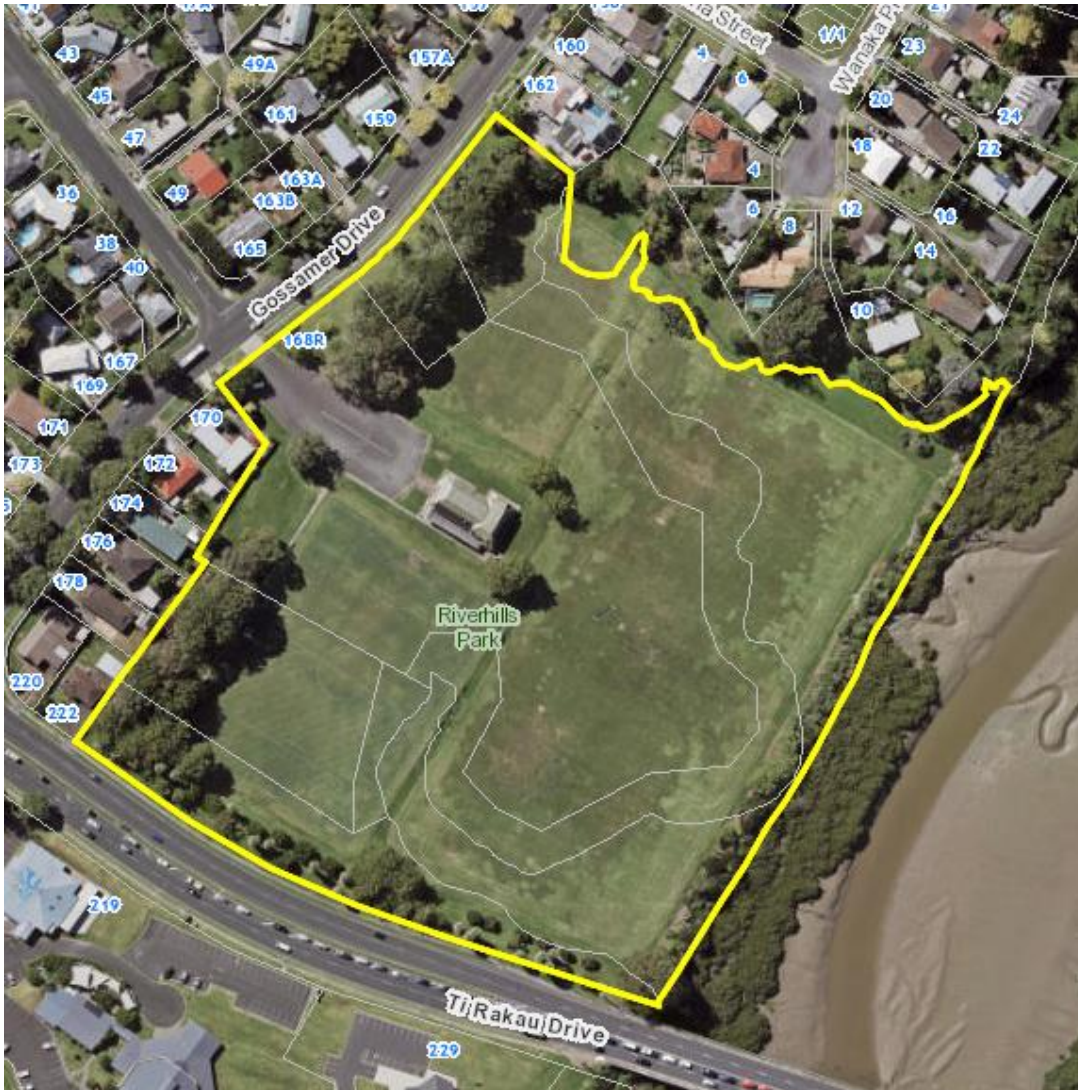
Figure 12. Riverhills Park (source Auckland Council Geomaps)
