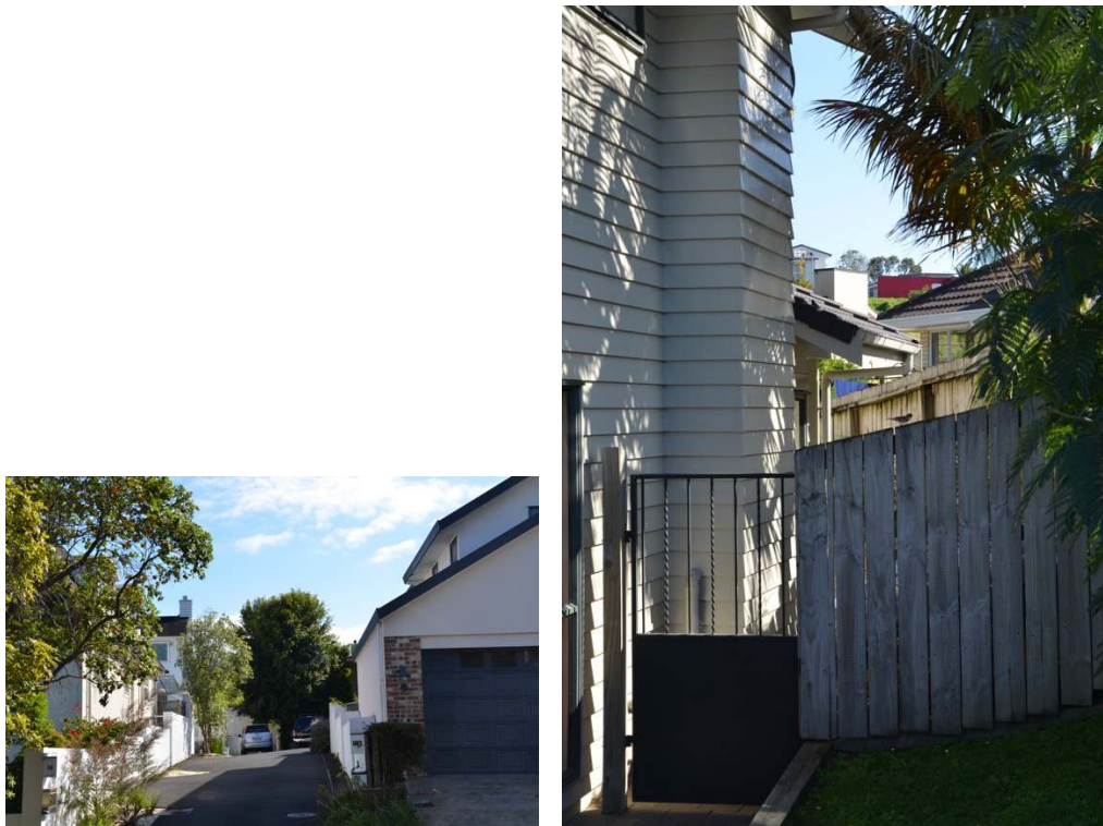
Figure 40: A typical view from John Rymer Place of the rear lots on the northern side of the street. These properties adjoin the southern boundary of the Site and accommodate houses which are very close together.
