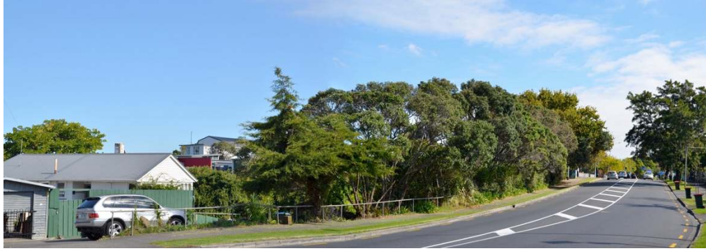
Figure 6: Viewpoint 1: The vegetated 223 Kohimarama Road boundary of the Site. One of the several Selwyn College buildings can be seen to the immediate right of the grey and gable roofed house on the left of the photograph. This house is at 245 Kohimarama Road and is owned by Selwyn College.
