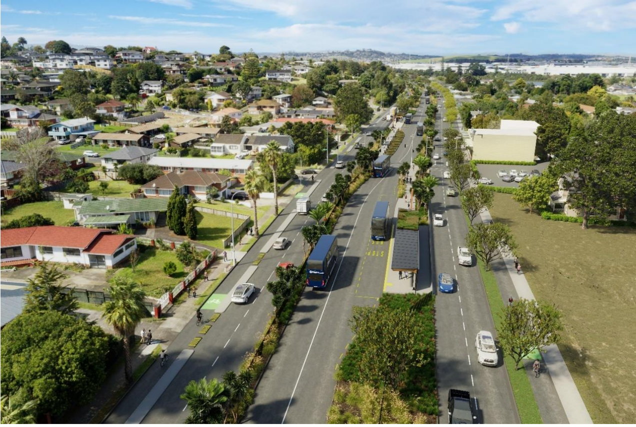
Figure 4: Artist impression of the busway and Edgewater Station on Ti Rakau Drive
