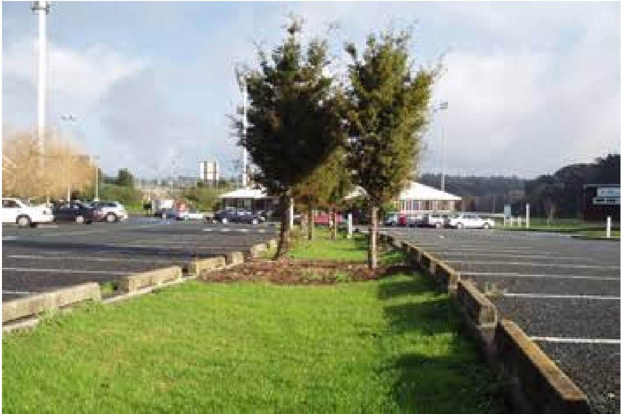
Figure 4: Example of a Swale (sourced from AC Swales and Filter Strips Construction Guide)
