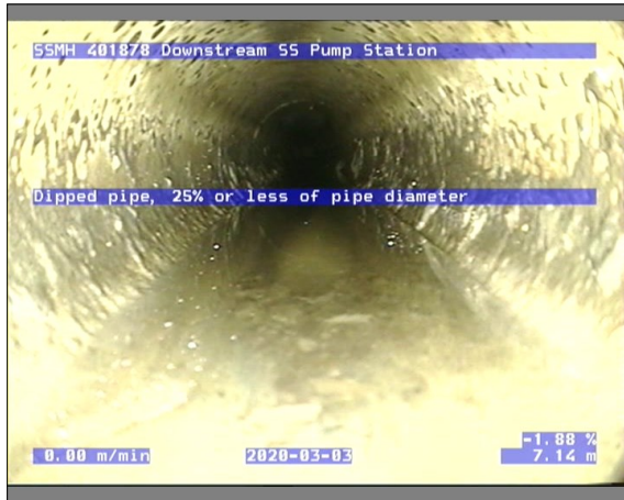
Photo: 3_3A 7.14m, Dipped pipe, 25% or less of pipe diameter
