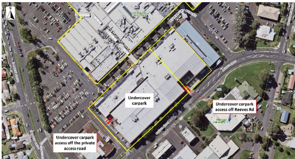
Figure 8 Pakuranga Plaza undercover carpark access during construction
