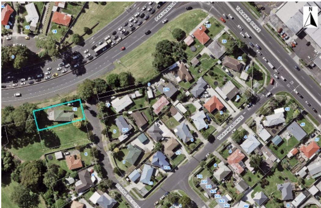
Figure 27 Satellite Compound at 12 Bolina Crescent
