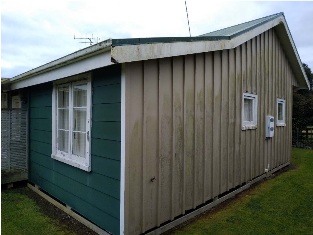
Figure 7-3: the pre-1940 cottage: another view.
