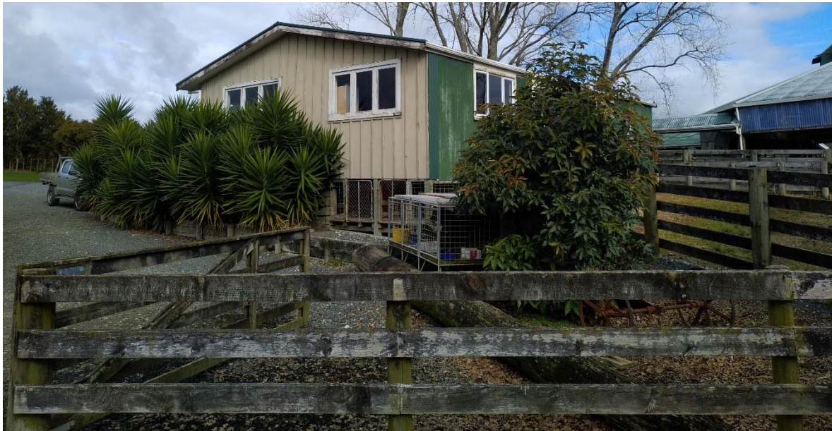
Figure 7-4: pre-1940 former shearing shed?
