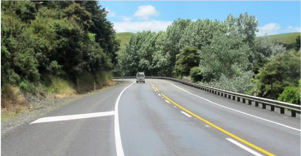
Photo 1 – Existing northbound approach to roundabout location
