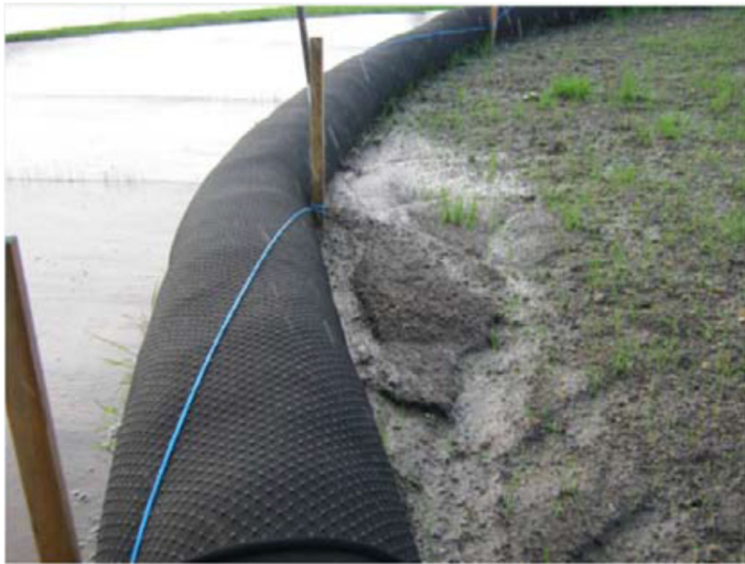
Figure 9 Silt or Filter Socks used as Edge Protection
