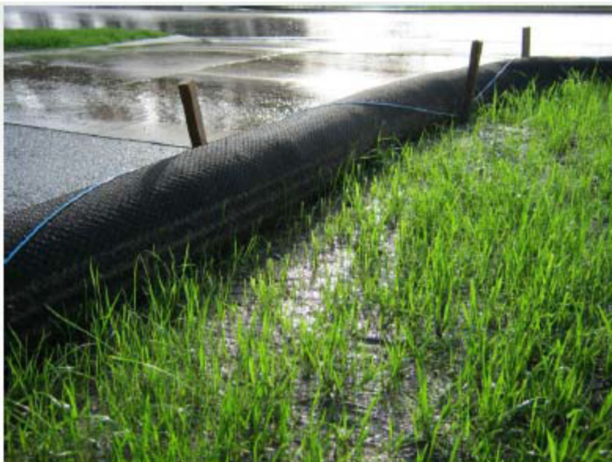
Figure 9 Silt or Filter Socks used as Edge Protection
