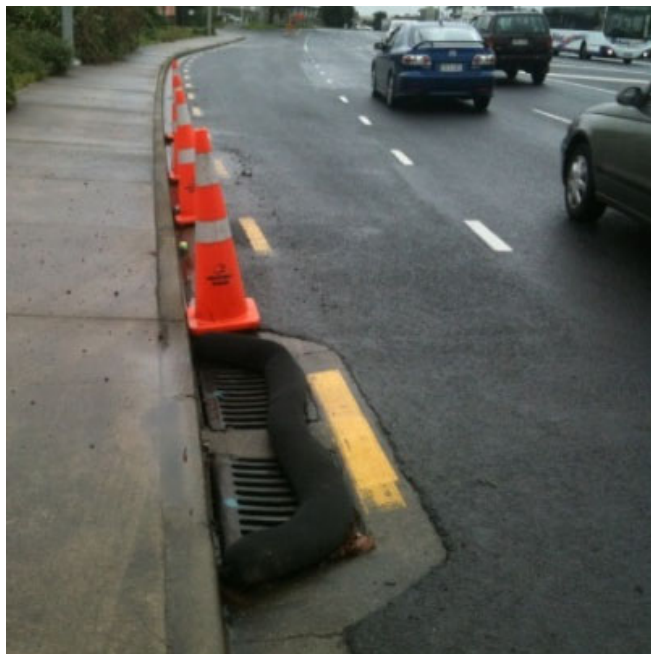
Figure 7 Example of Cesspit Protection
