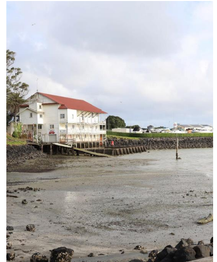
Figure 2.2: Takapuna Boating Club building with marina reclamation behind (Extract from Boffa Miskell VP-1)
