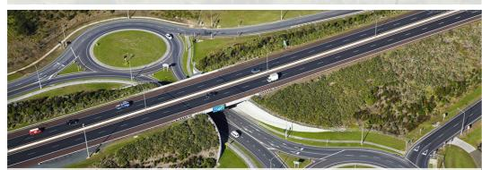
Figure 9: Interchange example: Similar with Te Hana and Wellsford on and off ramps connecting to roundabouts. Te Hana and Wellsford interchanges to have spill through abutments at the underpass (Refer to figure 16).
