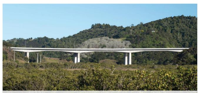
Figure 12: Waiwera River viaduct example of a good bridge design with no services visible, piers spanned to minimise impact on estuary and a slender super structure that uses light and shadow as design elements.
